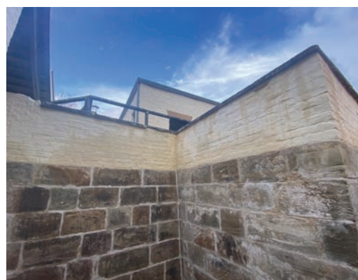
Below: Limewashing of brickwork and pointing stonework at Commandant's House Image: Pamela Hubert
