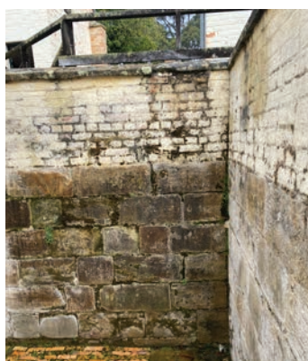
Below: Rear area of Commandant's House before limewashing and pointing Image: unknown
