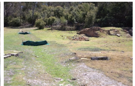
PHOTOGRAPH 2-23 DRAINAGE WORKS IN PROGRESS AT MAIN SETTLEMENT
