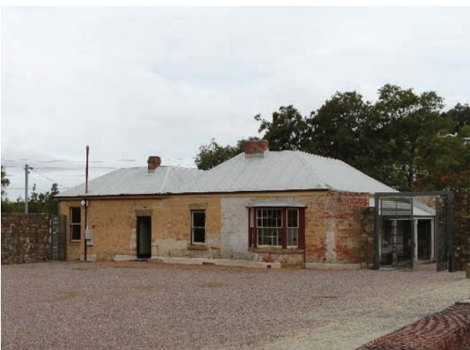
PHOTOGRAPH 2-10 MATRON'S COTTAGE YARD 4
