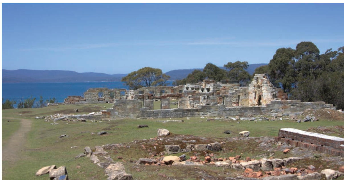
PHOTOGRAPH 2-3 VIEW LOOKING SOUTH-EAST ACROSS THE MAIN SETTLEMENT AREA OF THE COAL MINES HISTORIC SITE
