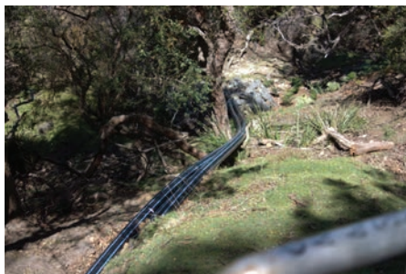
PHOTOGRAPH 2-22 DRAINAGE WORKS FROM MAIN SETTLEMENT DOWN TO THE WATERFRONT
