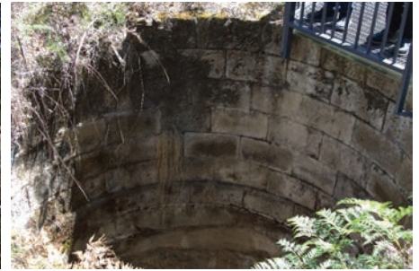
PHOTOGRAPH 2-14 BRICK LINED AIR SHAFT
