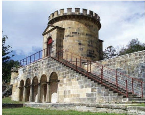
Port Arthur - Guard Tower DEPHA
