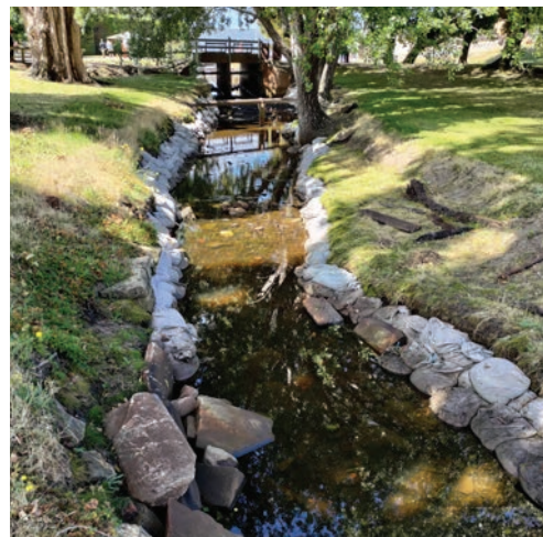
Sandbags used in Radcliffe Creek to reduce erosion during extreme weather events. Image: Dr Caitlin Vertigan
