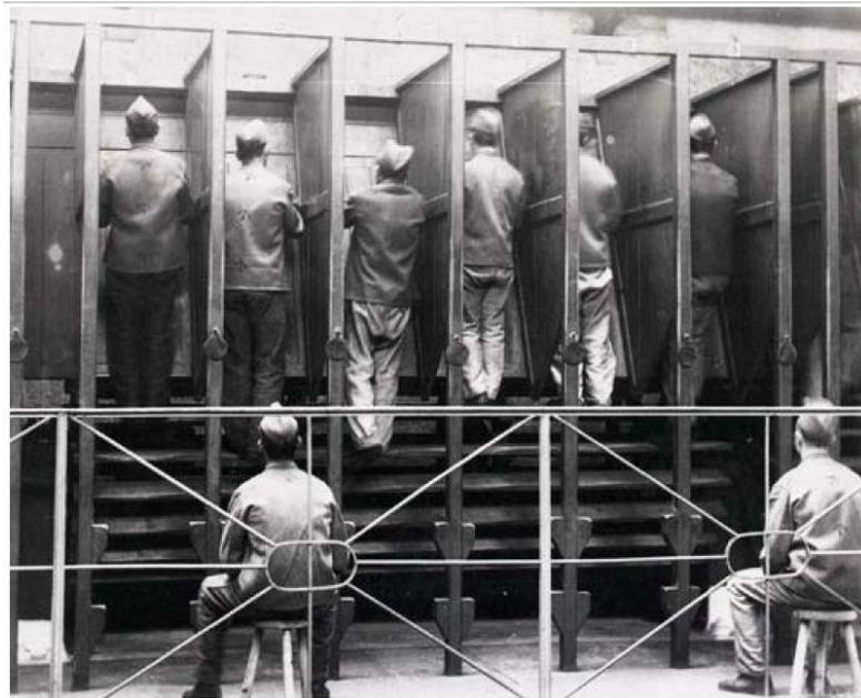
**Figure 13.** A treadwheel in operation at Pentonville Prison, London, 1895. The one at Port Arthur would have been similar. (Reproduced in Tierney, *Notes of Port Arthur's Tread Wheel*, 2009)
