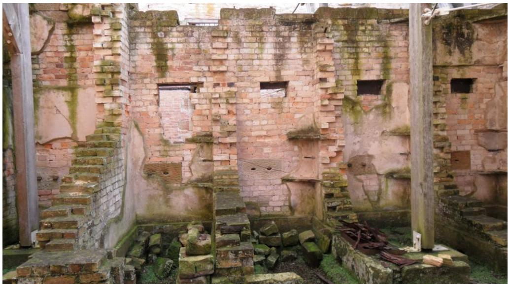
**Figure 54.** View of the remains of a number of cells with the foul air egress vent in the rear wall [authors 2010]
