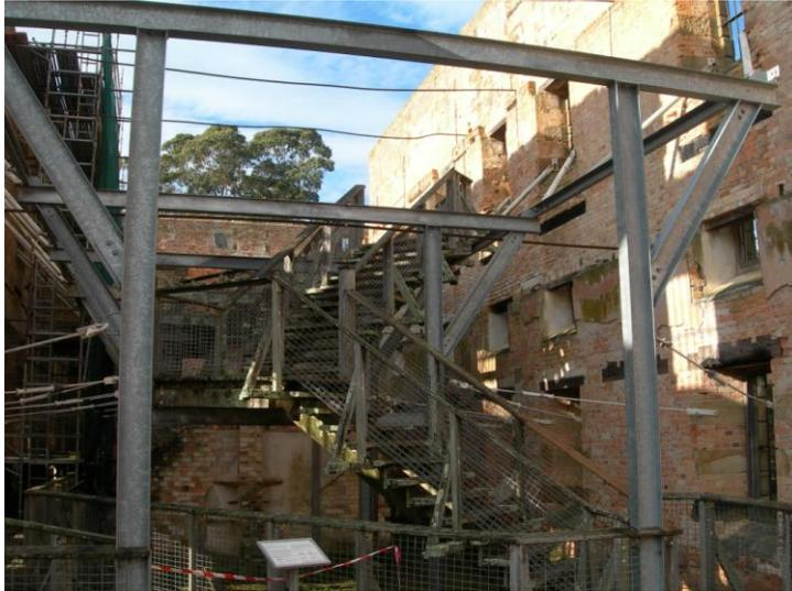
**Figure 55.** Interior view of the Penitentiary ruin structural stabilization infrastructure and walkway. [authors 2010]
