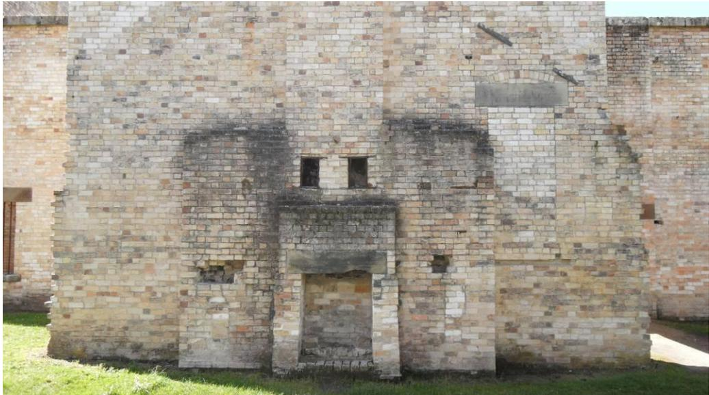
**Figure 25.** *The surviving north wall of the Laundry. The fireplace for boiling water is at centre, ground level. To the right is an elevated doorway (indicated by a stone lintel), now bricked in. (Andronas Architecture, 2010)*
