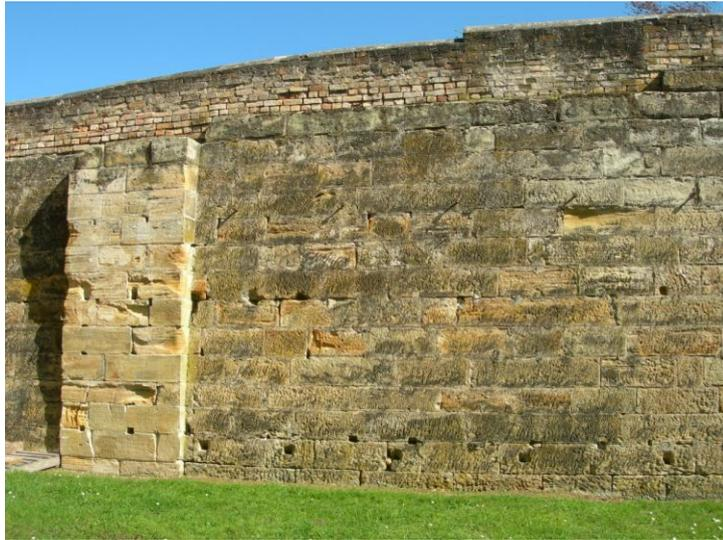
**Figure 70.** Stone pier which originally supported the water wheel flume [authors 2010]
