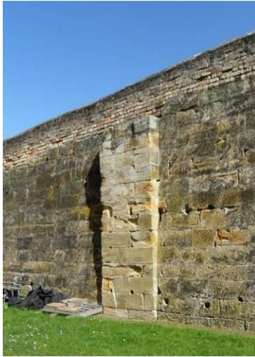
**Figure 8.** Left: Base of the flume pillar in the Champ Street retaining wall enclosing the rear wall of the Penitentiary (Andronas Conservation Architecture, 2010).
