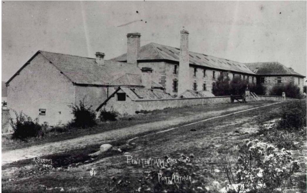
**Figure 26.** View of the Laundry and Bakehouse from Champ Street, looking north-east, after 1864 when the laundry and kitchen digester boiler was installed (note its free-standing chimney). Note the small, hipped-roof structure linking the two building – this may have been the drying room. (PAHSMA ref 66-1030)
