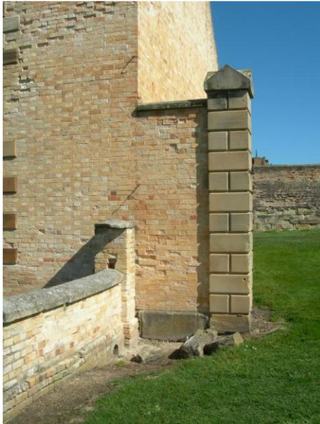
**Figure 75.** Section of masonry wall and stone pillar originally providing access to the workshops yard [authors 2010]
