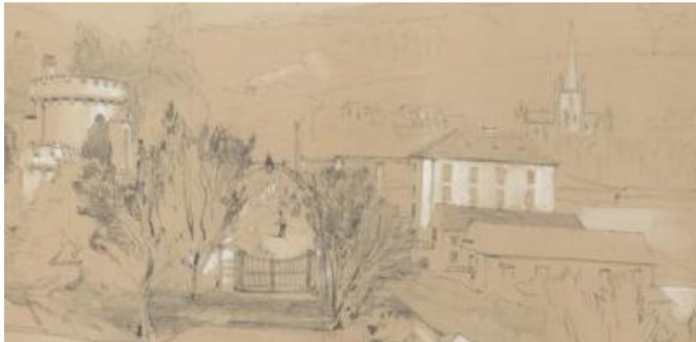
**Figure 7.** Detail from John S Prout's sketch 'The settlement, Port Arthur, V.D.L., from the commandant's residence, May 20, 1845', showing (from left to right) the siphon rising up south of Champ Street, and two support pillars (on either side of Champ Street) supporting the flume which then enters the Flour Mill at eaves level. (National Library of Australia, nla.pic-an2479033)
