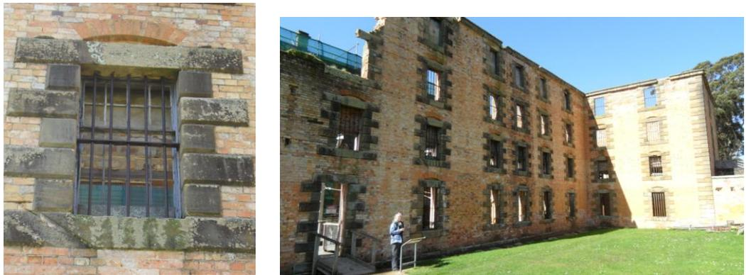
**Figure 52.** View of a southern window with timber framed window, masonry infill behind and metal bars in front (left image) and general view of the south wall of the Penitentiary ruin (right image) [authors 2010]
